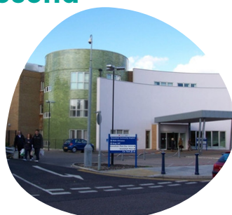
Gravesham Community Hospital Gravesend
